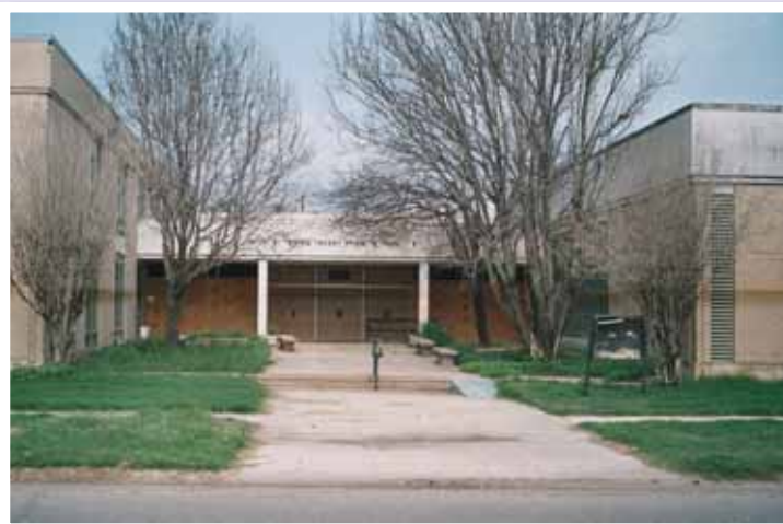
Beth Israel synagogue in New Orleans was heavily damaged by Hurricane Katrina, with ten feet of water flooding the shul and destroying Torahs and sefarim. Courtesy Beth Israel
